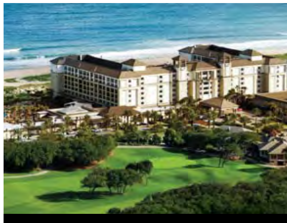
A SPECTACULAR 444-ROOM RESORT HOTEL, THE RITZ-CARLTON, AMELIA ISLAND IS A SEASIDE RETREAT FOR NATURE LOVERS AND THOSE WHO THRIVE ON AN ABUNDANCE OF SUN, SAND AND OUTDOOR SPORTS. THE PROPERTY RECENTLY INSTALLED AN AQUARECYCLE SYSTEM THAT RECLAIMS AND REUSES LAUNDRY WASTEWATER HELPING BOTH THE ENVIRONMENT AND THE BOTTOM LINE.
