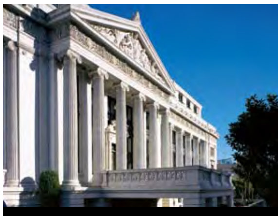
THE RITZ-CARLTON, SAN FRANCISCO IS A LANDMARK IN THIS GATEWAY TO THE PACIFIC. A RECENT RENOVATION INCLUDED THE INSTALLATION OF A MICROTURBINE COGENERATION PLANT THAT SAVES ENOUGH ELECTRICITY TO POWER 200 AMERICAN HOUSEHOLDS AND REDUCES EMISSIONS BY 800 TONS OF CO 2 PER YEAR.
